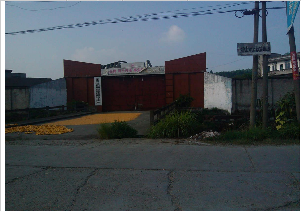
Evidence 11 – Yuegou facility main gate with corn drying under the sun
